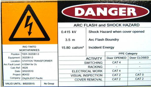
Fig. 1 Arc flash label sample
