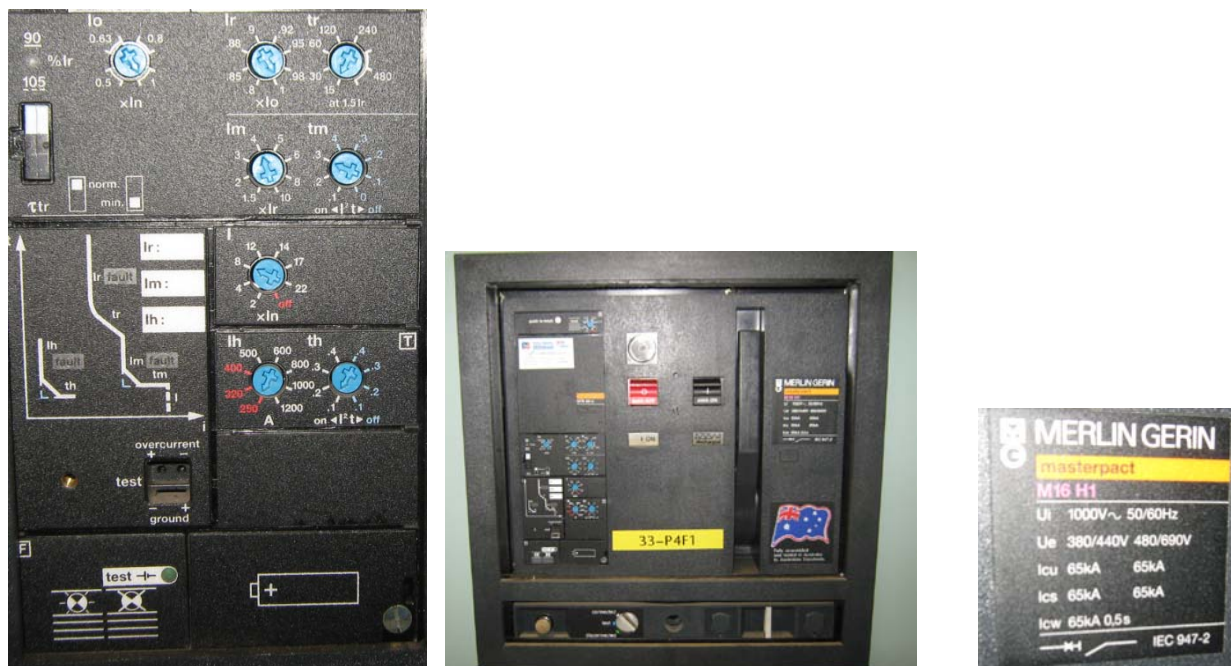
Figure 5 – Merlin Gerin Masterpact ACB 1600A H1 3-pole fitted with STR 58U trip unit no GF
